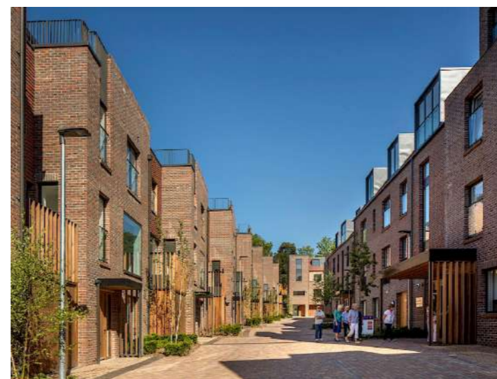
Varied roofline and use of roof terraces gives harmonious variety to the street, Woodside Square, London, Pollard Thomas Edwards
