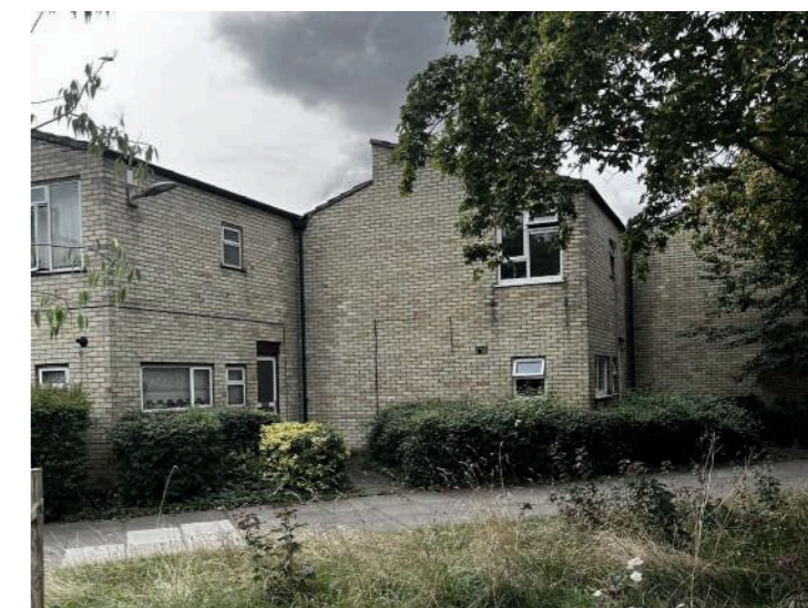
6. Front Elevation of a typical Nuns Way facing on to a green open space
