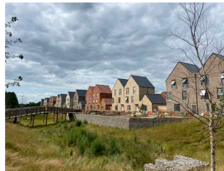
Houses looking over landscape with SUDs. Services hidden away at the rear. Marleigh, Pollard Thomas Edwards
