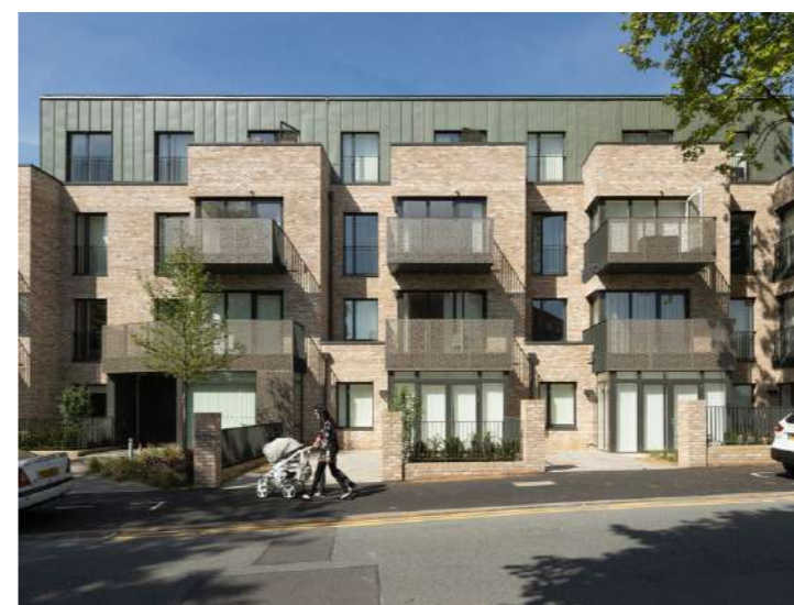
Balconies for all upper floor flats, Colby Lodge, Pollard Thomas Edwards
