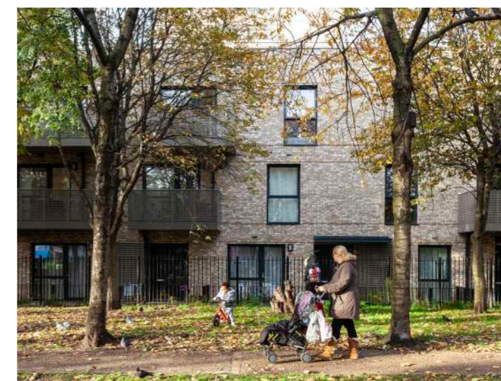
Improving existing unattractive links, King Square, London Borough of Islington , Pollard Thomas Edwards
