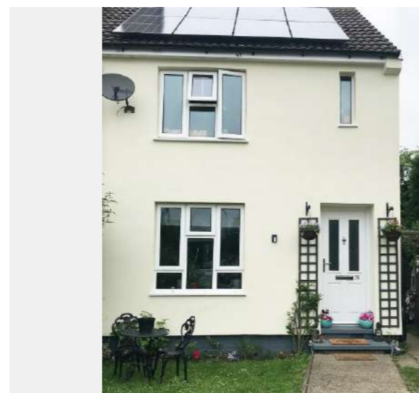
Insulated render retrofit project, Cambridge City Council Design Code, February 2024
