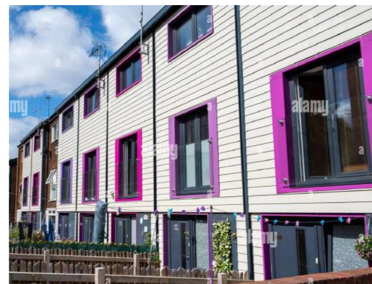
Overcladding with boarding to meet "energiesprong" standards, Nottingham, Richard Partington Architects
